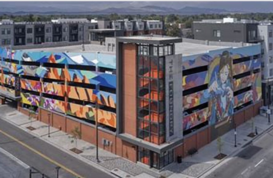
The Loveland Foundry Parking Structure | 255 E. 2nd St., Loveland, CO
